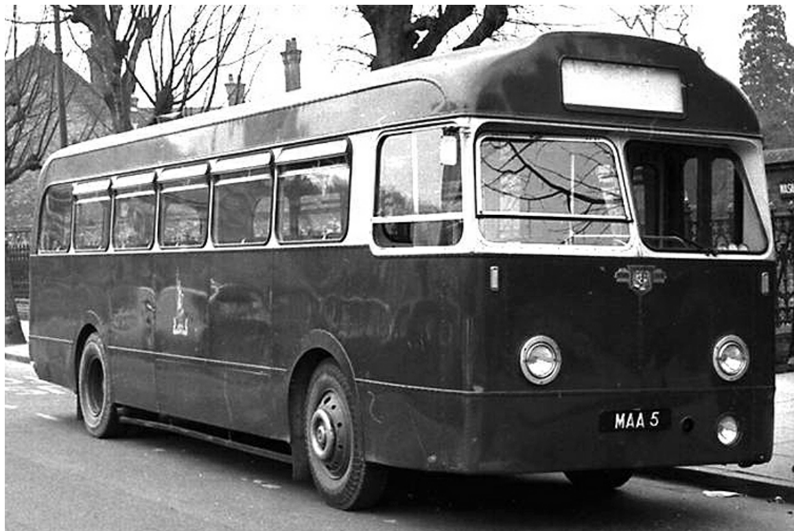
1953 Leyland PSUC1/1T MAA5 with Weymann BET-style 44-seat bus bodywork. This bus was withdrawn in 1965. (John Boylett courtesy John Kaye).
